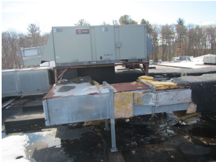
Damaged ductwork for rooftop AHU
