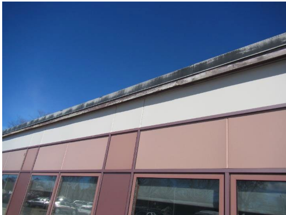
Damaged wooden trim and eaves at the top of the building edge
