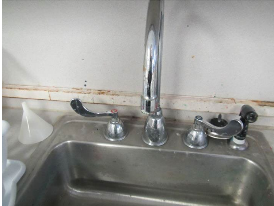
Water-damaged backsplash on a classroom sink
