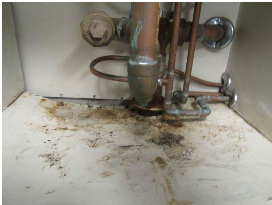
Water-damaged, rusted, and bent material underneath a classroom sink
