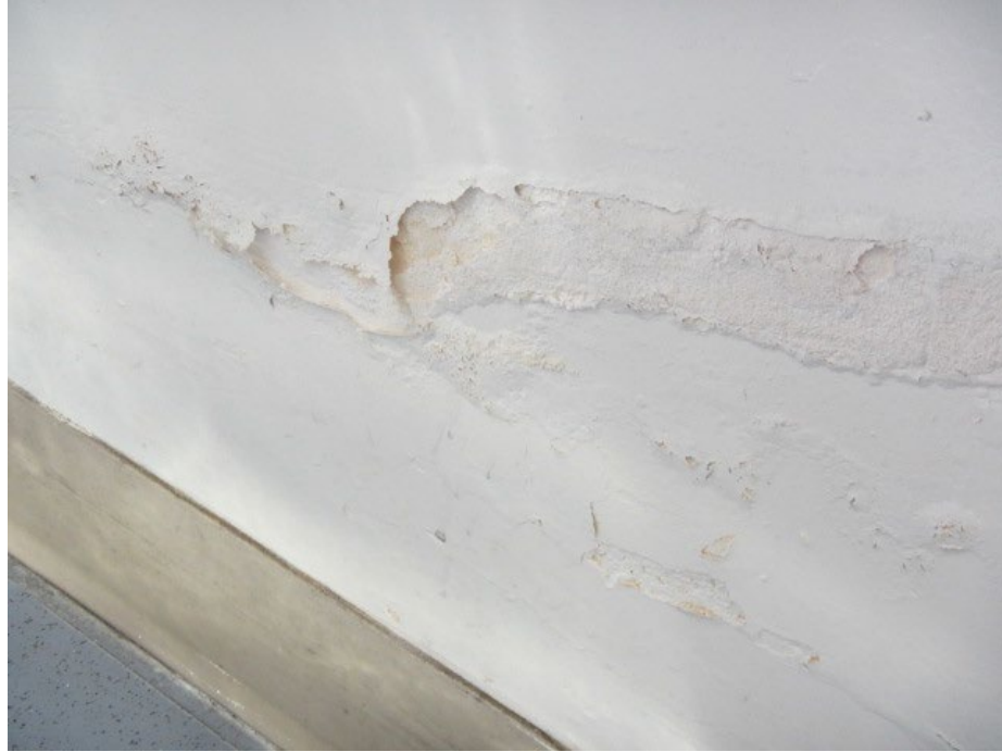
Water-damaged plaster
