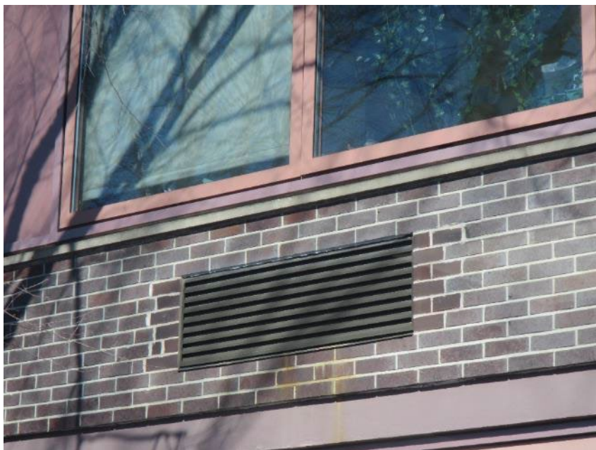
Univent vent on the outside of the building
