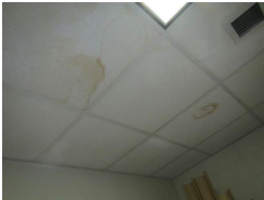
Water-damaged ceiling tiles
