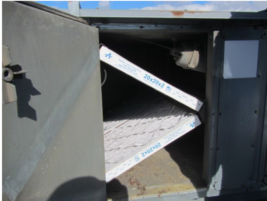
MERV 13 filter in rooftop AHU
