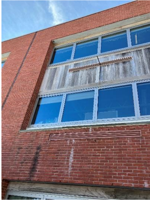
Water damage and stains on brickwork
