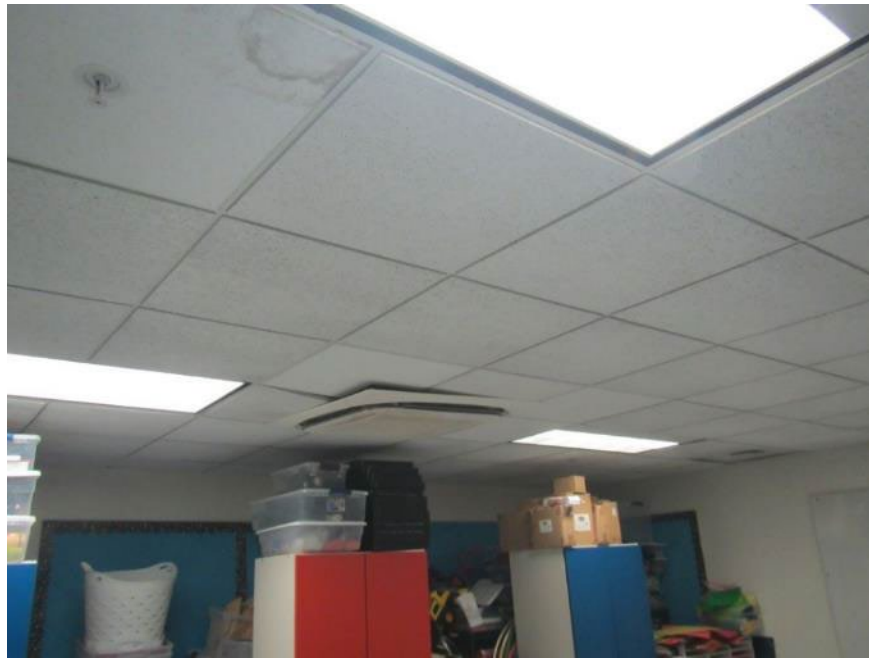
items piled near ceiling and supply vent
