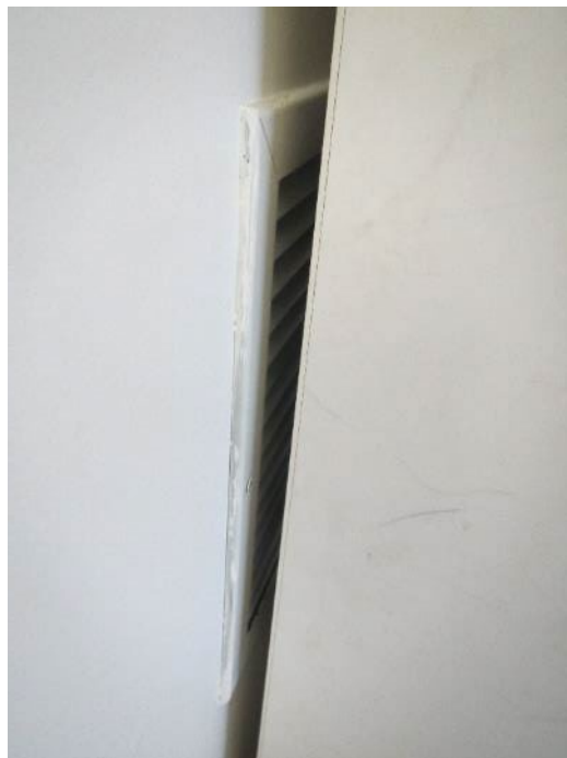
Exhaust vent blocked by a cabinet
