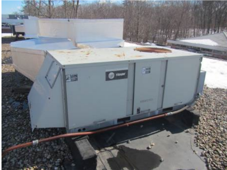
Air handing unit on the roof
