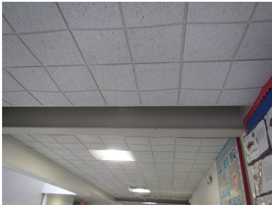
Bowing ceiling tiles in a hallway
