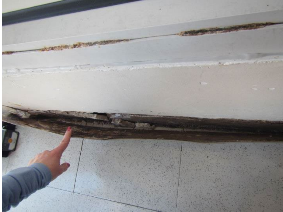
Water-damaged wall on the lower level
