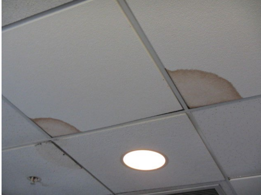
Water-damaged ceiling tiles
