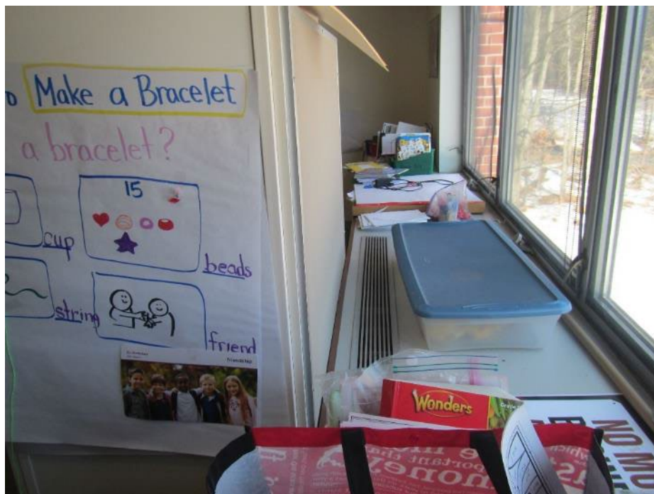
Univent (on the right side of picture) blocked by furniture
