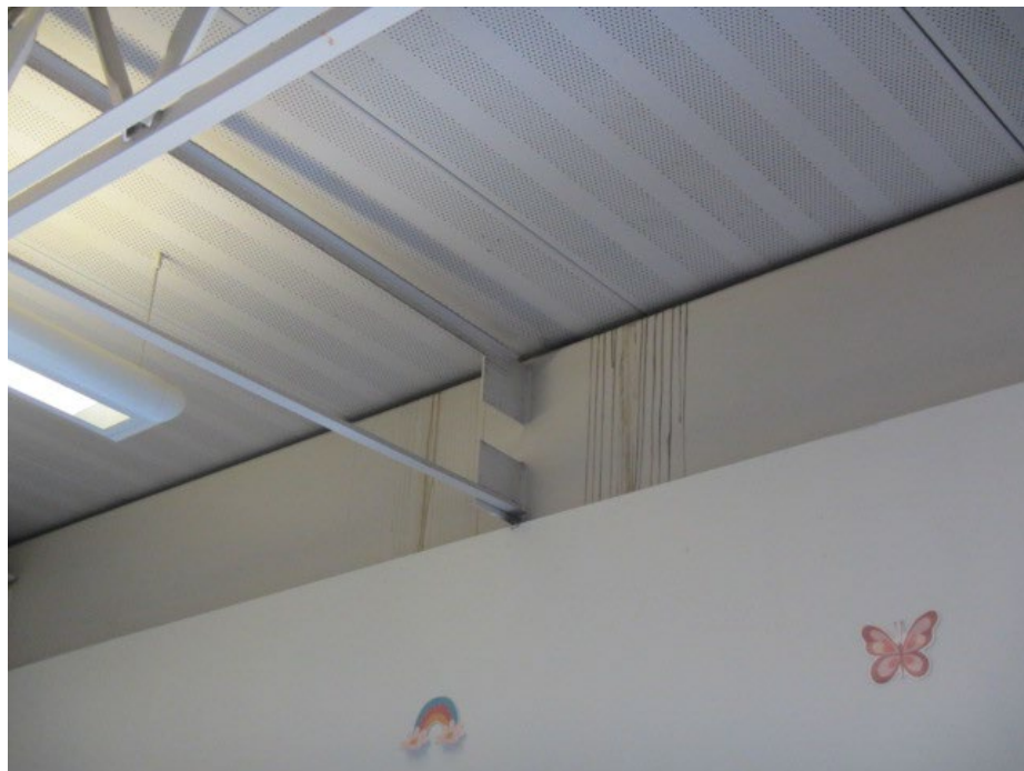
Staining from roof leak on wall in room 203
