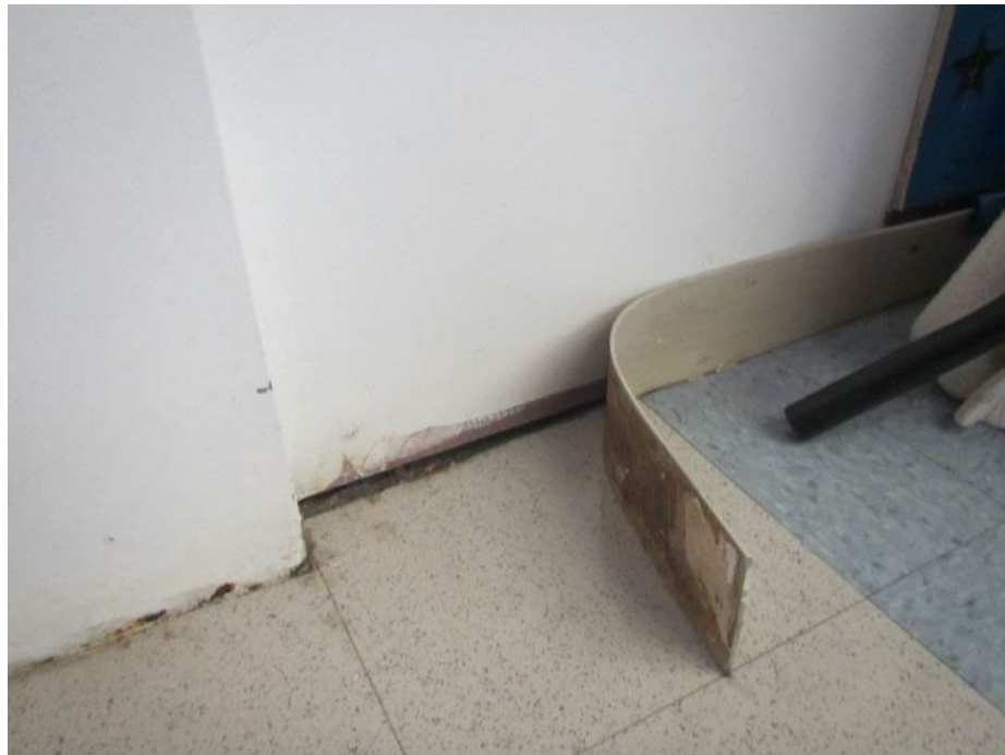
Water-damaged wall and loose coving on the lower level
