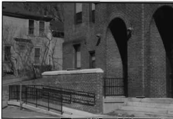
Universal access to the Central School (1904/24; 10 Ditson Pl.) is neatly provided at one of its major entrances. A brick wall conceals the upper ramp, repeating the materials and planar forms of the building and minimizing the more cluttered effect of lengthy railings.
